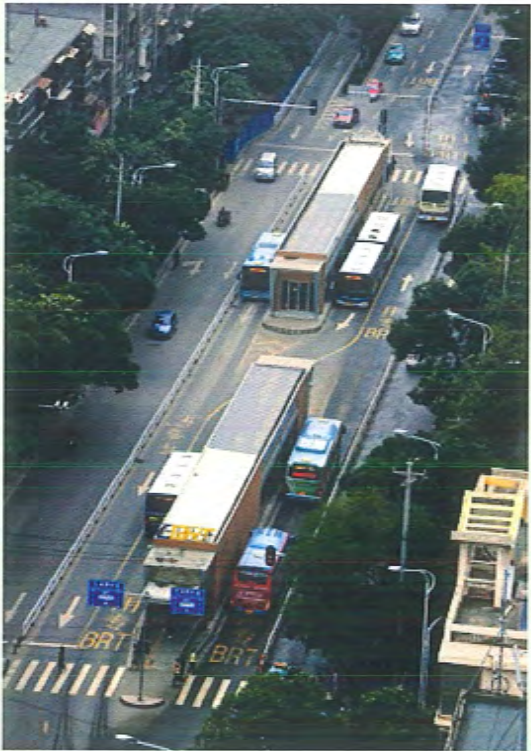
The Lanzhou BRT system has center stations that only serve one direction of travel.
