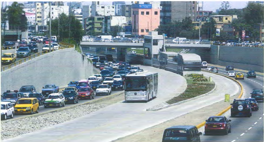
Lima, Peru, uses reinforced concrete over its entire busway.
