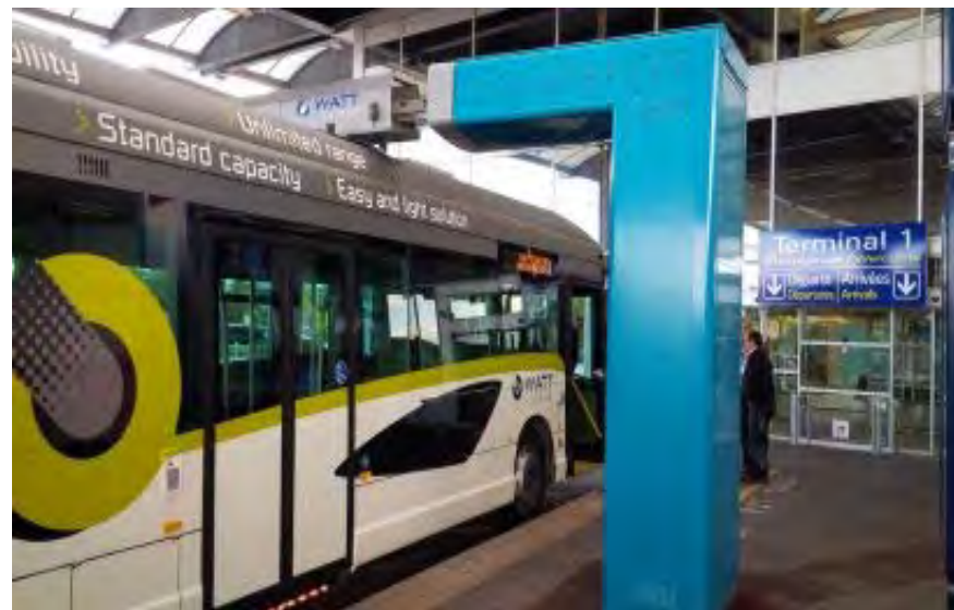
Photo 3.5 Station de recharge PVI
